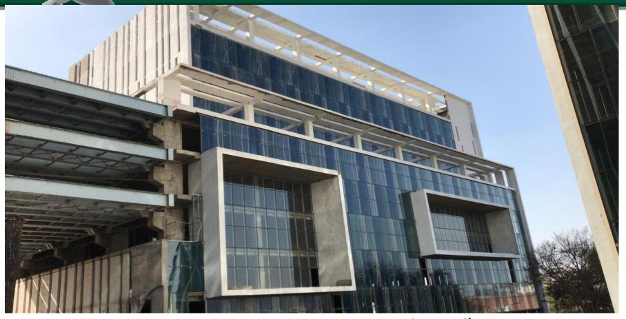
Curtain glazing aluminum glass 1<sup>st</sup> to 5<sup>th</sup> floor 98% complete. 6<sup>th</sup> and 9<sup>th</sup> floor interior fit out work is on progress
