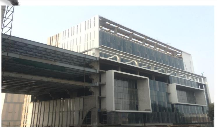
Curtain glazing aluminum glass 1<sup>st</sup> to 5<sup>th</sup> floor 80% complete. External Painting work is on progress.
