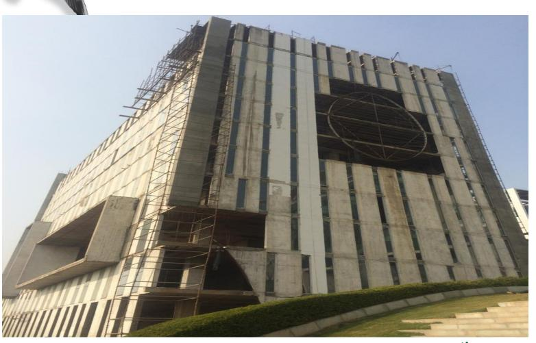
East side Slit window glass fixing up to 10<sup>th</sup> floor complete. External painting work is on progress.
