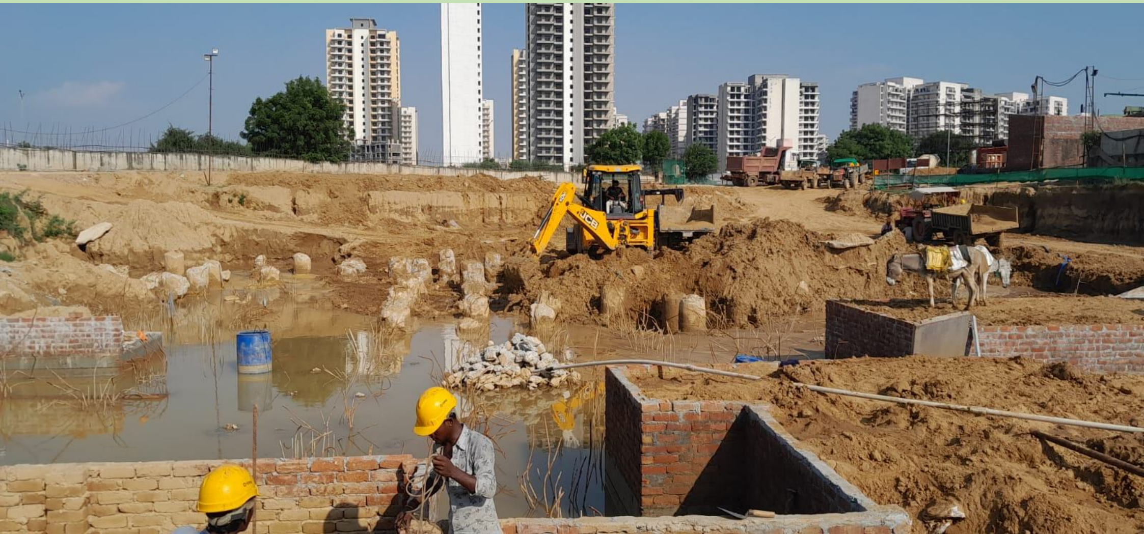
TOWER-2. Excavation for raft complete
