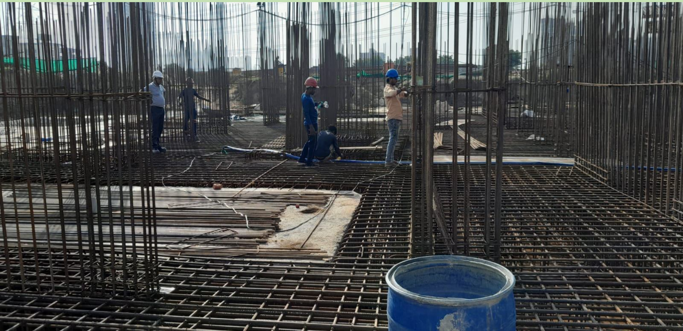
TOWER-3. RAFT WIP
