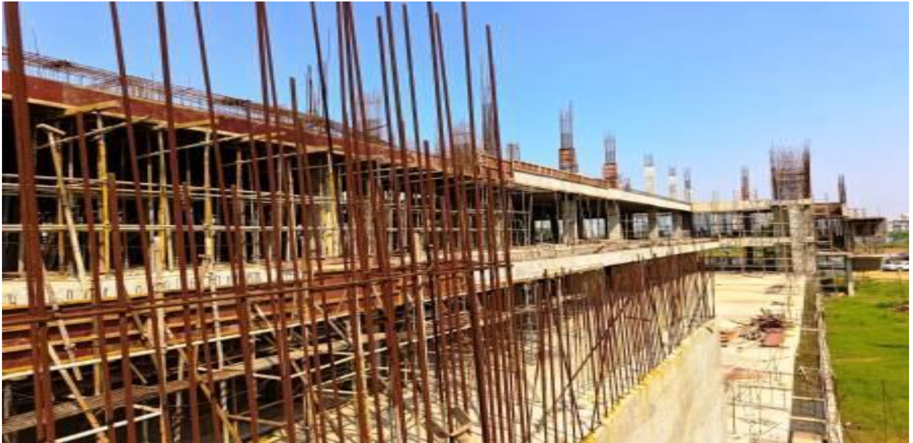
SF roof column casting in progress (Elevation B)
