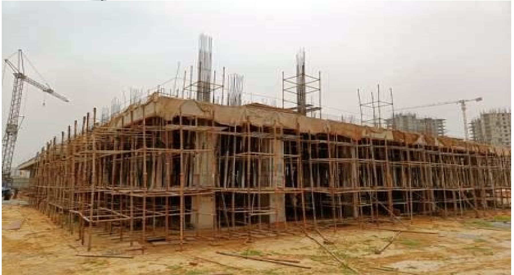
FF roof slab casting in progress (Elevation B)
