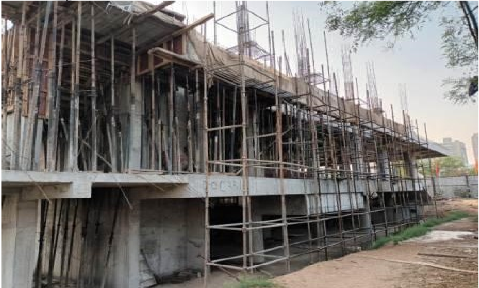
FF slab casting completed
