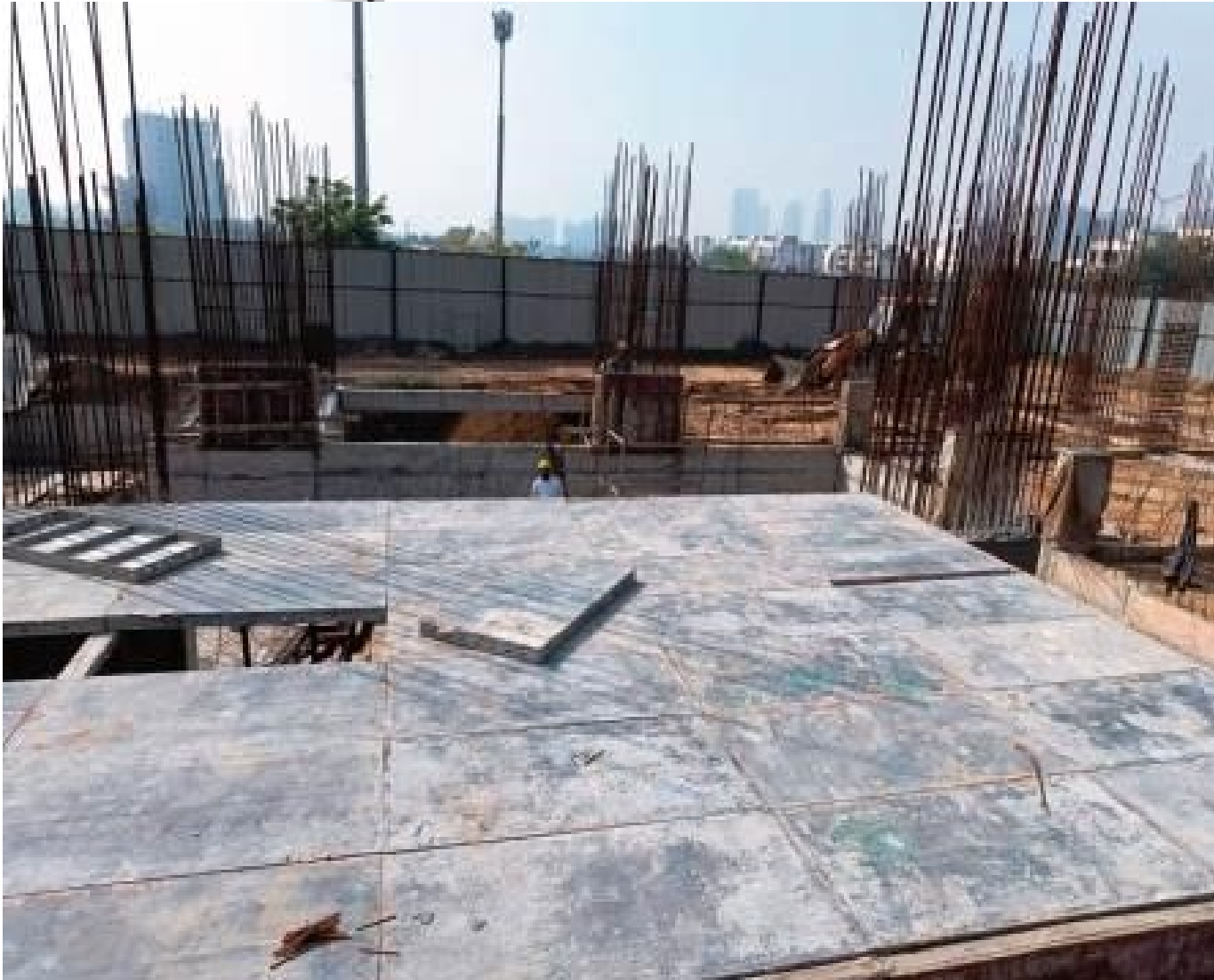
Stilt Roof Slab Shuttering work In Progress
