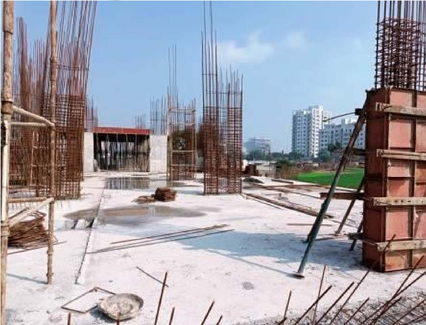
Casting of GF slab completed
