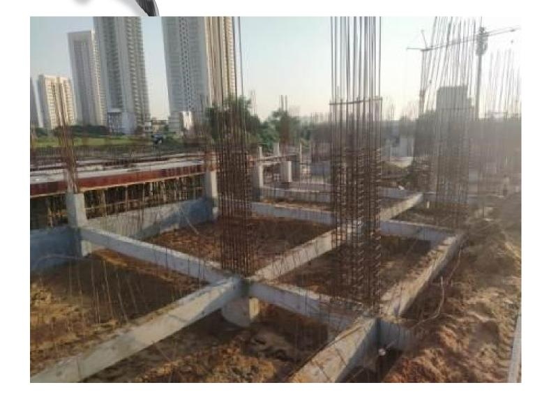
Casting of plinth beam completed
