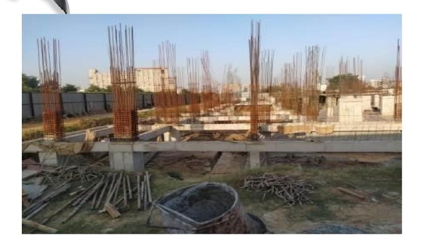
Column Reinforcement work is on progress.
