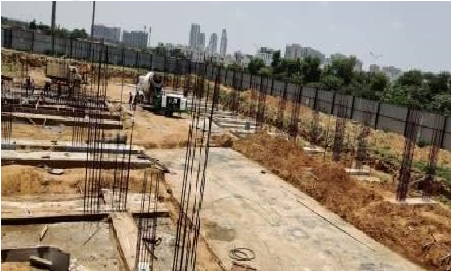
Casting of Column Raft
