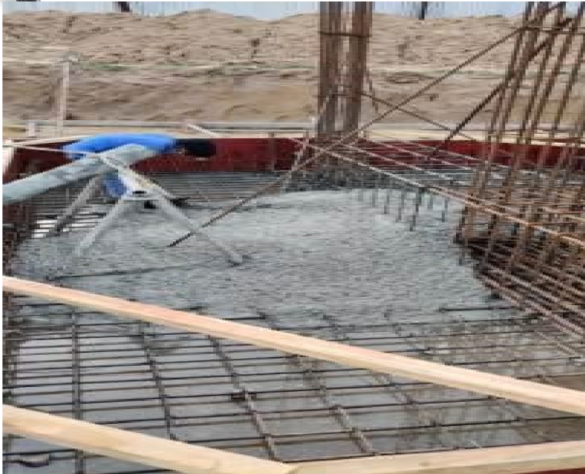
Raft work is on progress.
