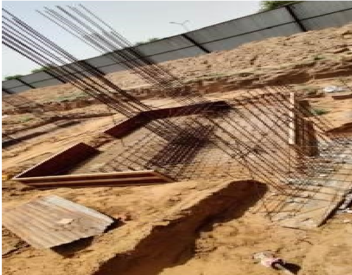
Reinforcement Work of column in Progress
