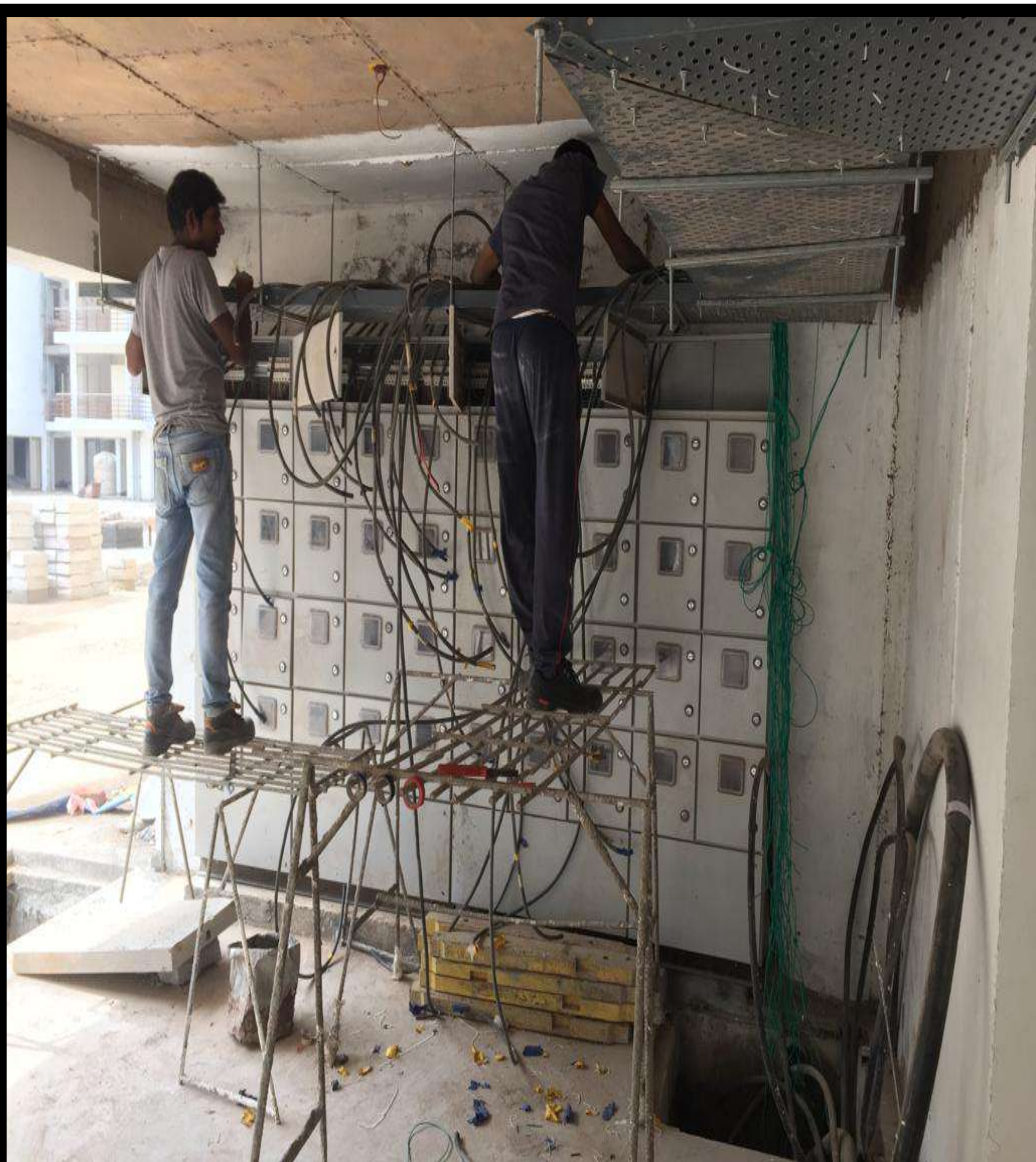
Sub Main Meter Board Termination Work is in progress
