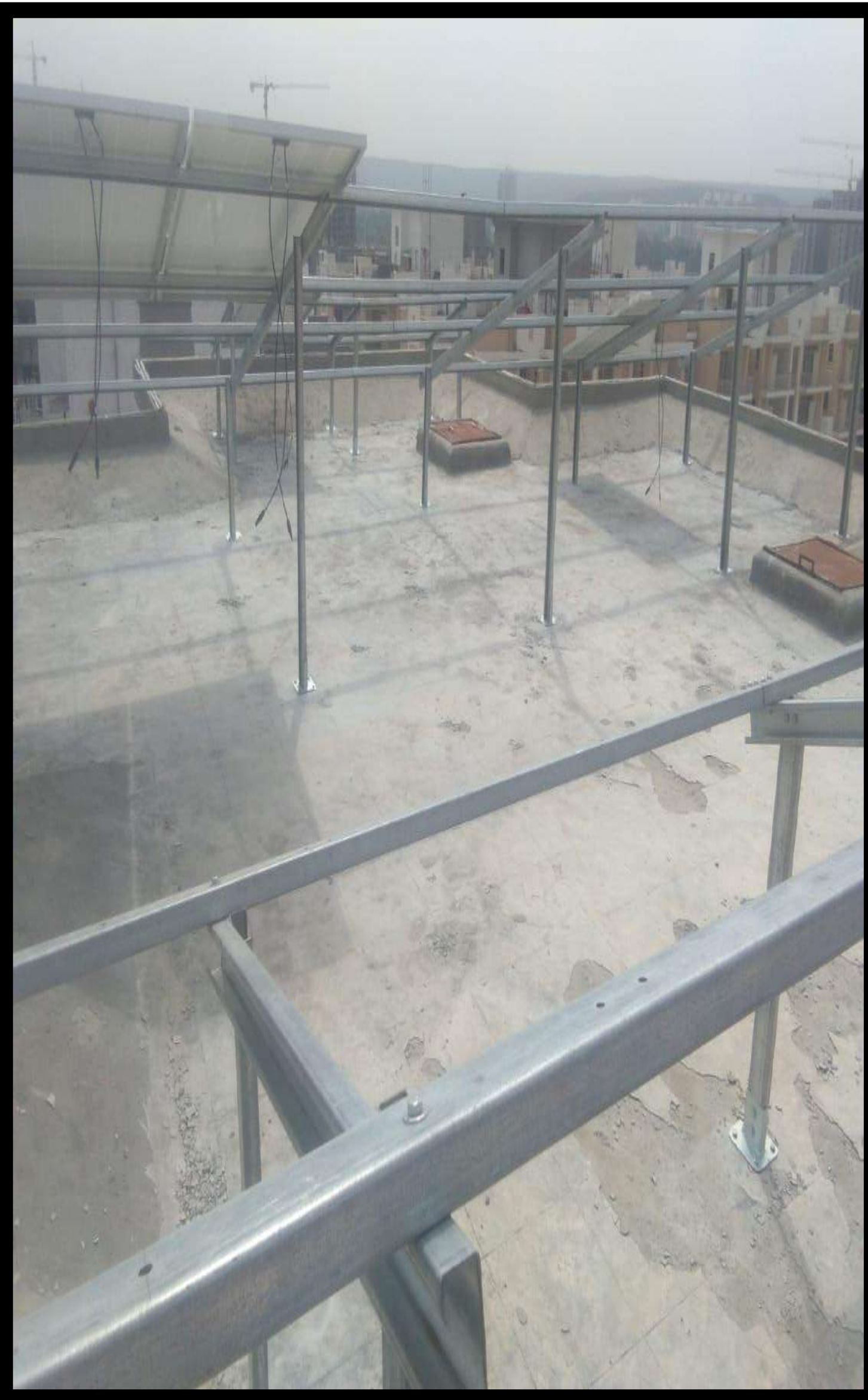
Solar Panel Framing Work – Tower – 15 & 16
