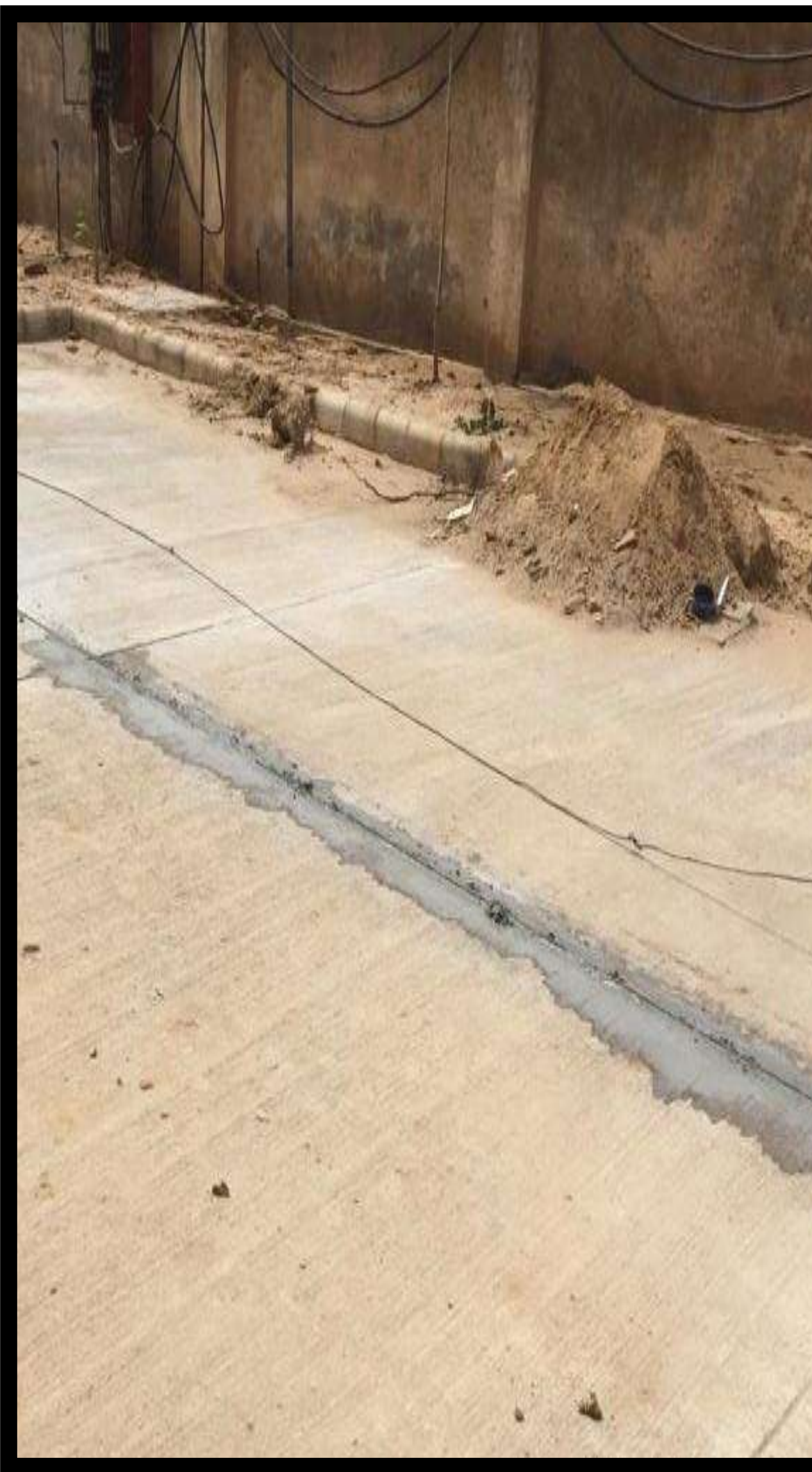
Groove Cutting Work is in progress
