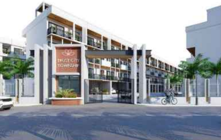
PROJECT MANAGEMENT CONSULTANCY
