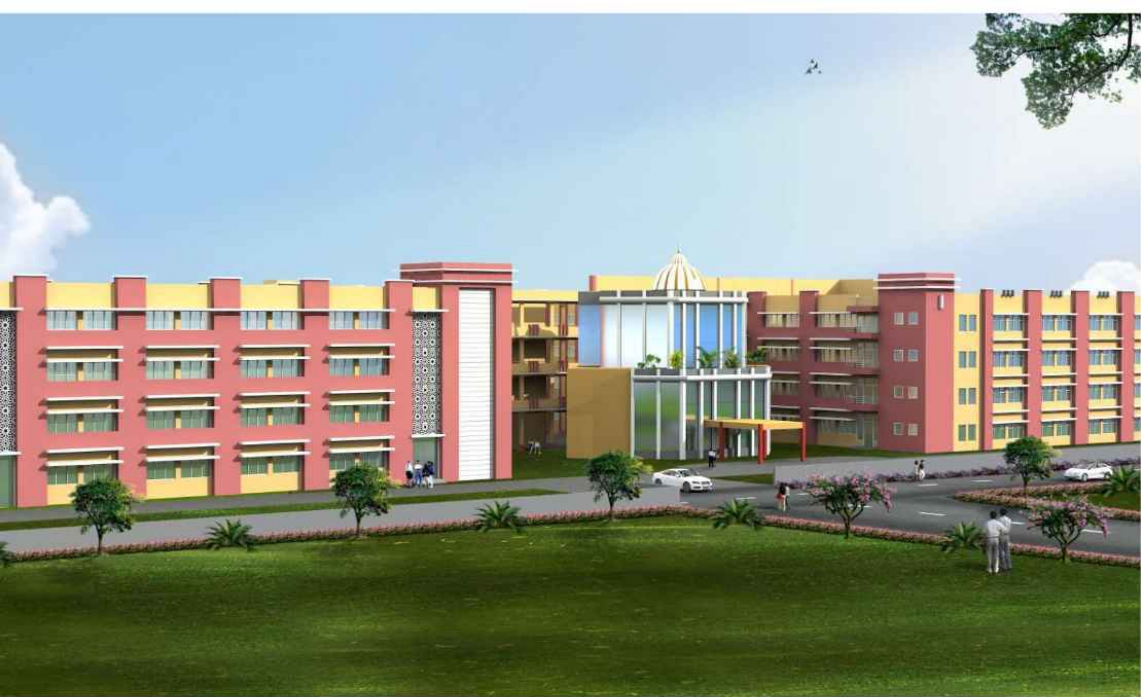
SENIOR SECONDARY SCHOOL BUILDING AT VILL DHARAMPUR, GGN FOR M/S PROGRESSIVE CHARITABLE TRUST (THE SHIKSHIYAN SCHOOL)
