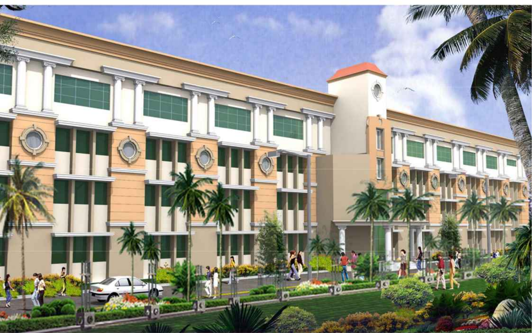
INSTITUTE BUILDING (B.ED COLLEGE), VILL. TIKRI, GURGAON FOR M/S CH. PRATAP SINGH MEMORIAL TRUST
